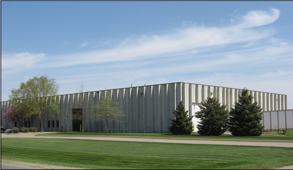
South / West side of building showing 2 drive in doors (1 each side)
